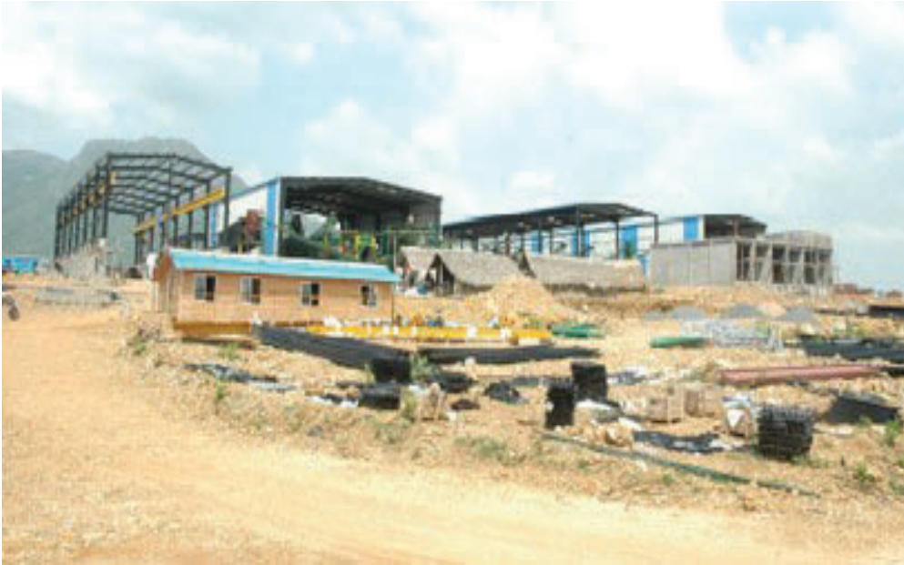
Figure 69: New site of SWM in Chettichavadi
