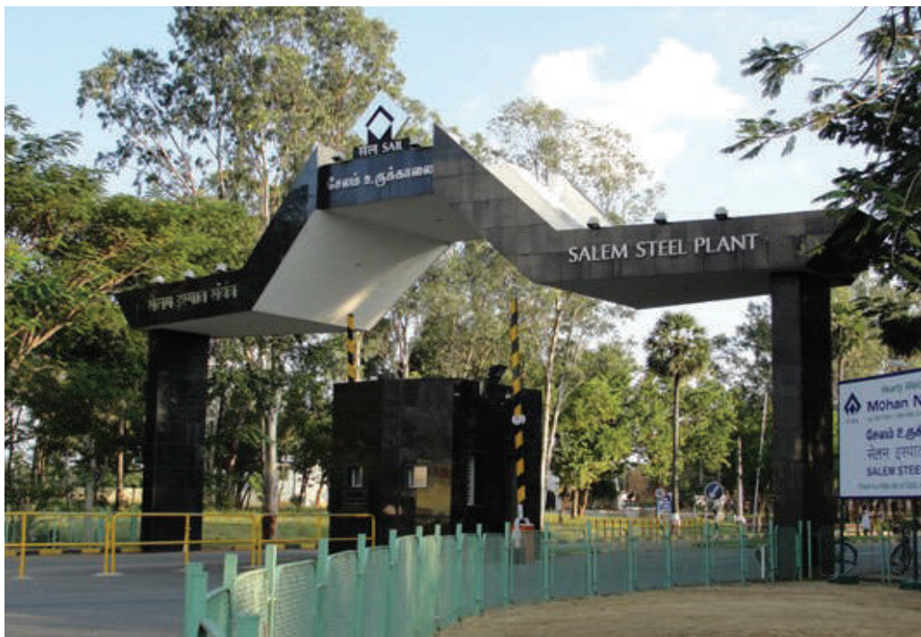
Figure 6: Salem Steel plant
