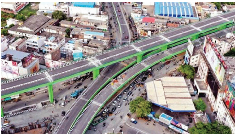
Figure 16: Salem Double decker Flyover
